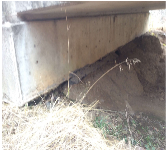
PHOTO 2 Description Bent 5 settlement in the compacted embankment.
