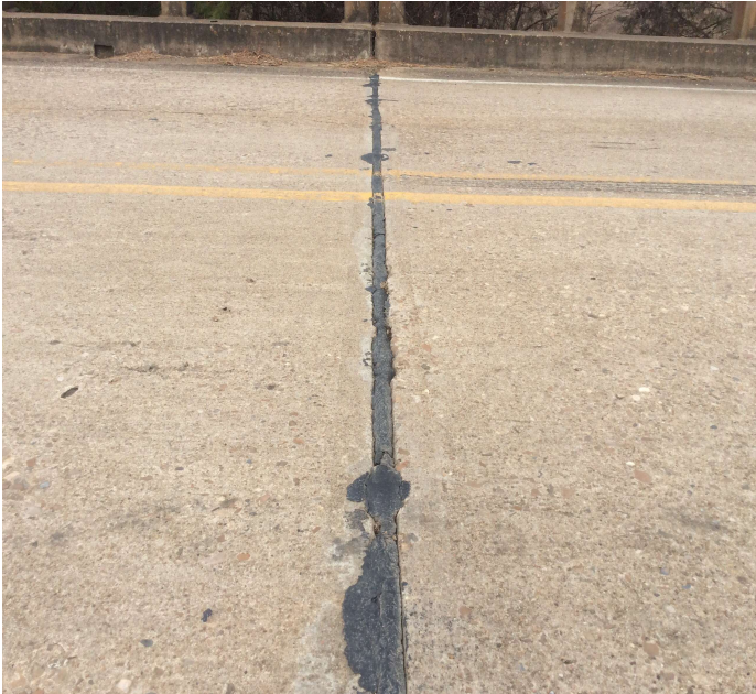
PHOTO 3 Description Deck joint sealant has deterioration and leaks water onto the substructure caps. Bent 4 pictured.
