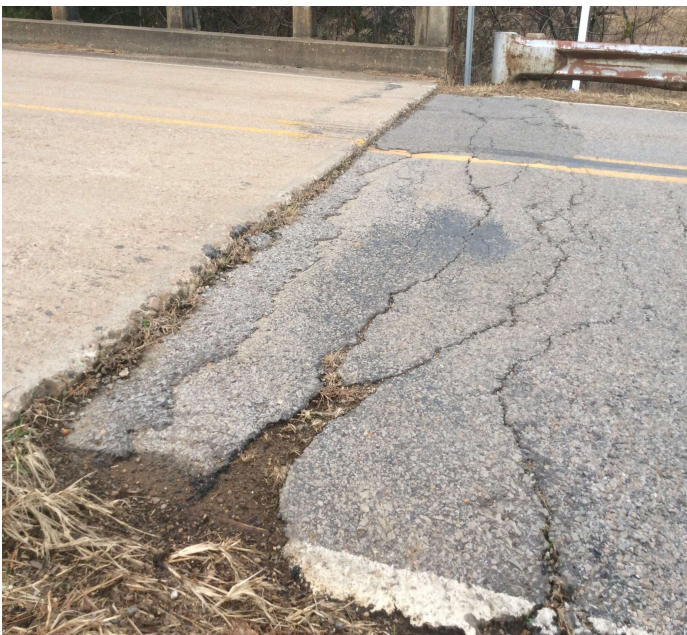
PHOTO 1 Description Approach Roadway Settlement in the East approach.
