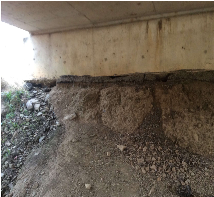
PHOTO 1 Description There is minor earth settlement under the East abutment with asphalt placed in some of the voids as a type of repair.
