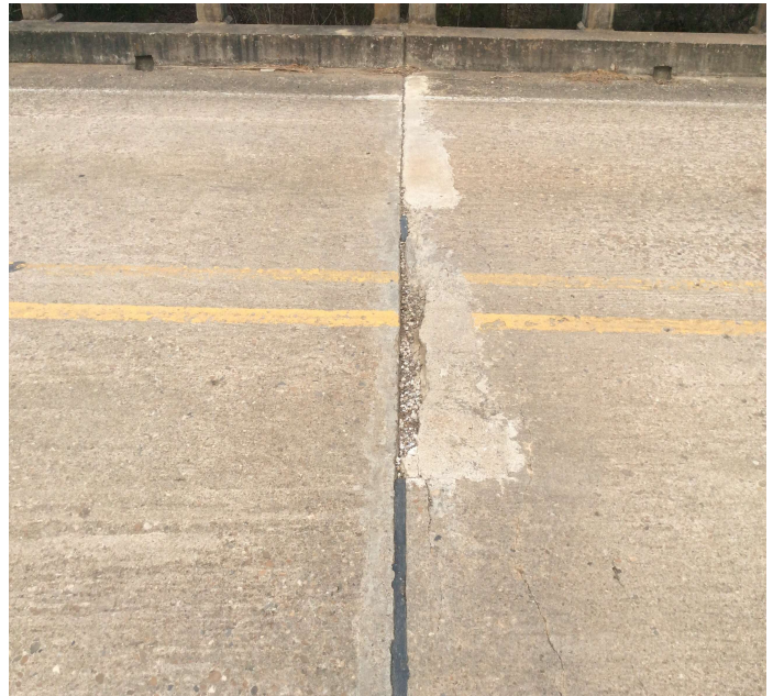
PHOTO 2 Description Deck joint sealant has deterioration and leaks water onto the substructure caps. Bent 3 pictured.
