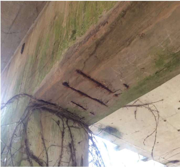
PHOTO 1 Description Shallow spalling with exposed reinforcing steel (Stirrups) visible from the undersurface of Bent 2 cap. Exposed reinforcing steel has very little concrete cover from the construction process with initial section loss typical.
