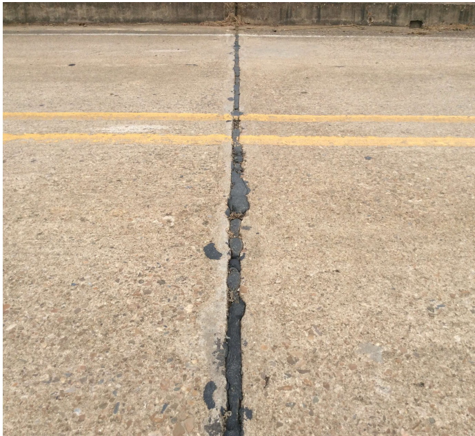
PHOTO 1 Description Deck joint sealant has deterioration and leaks water onto the substructure caps. Bent 2 pictured.
